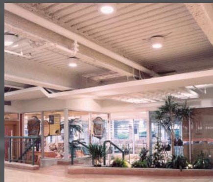
Southwest Fireproofing Type 5GP on steel beams & decking
